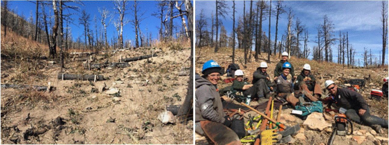
Log Erosion Barriers - MHYC
