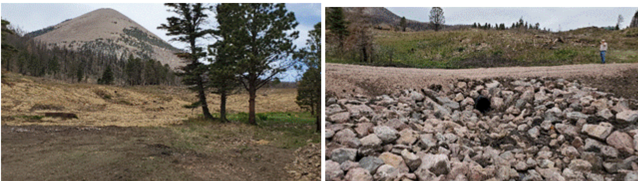
NRCS – Central Valley: Mulch and Seed (left), Elk Road Armored Crossing (right)
