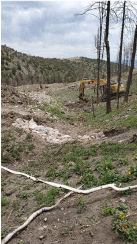
NRCS – West Valley: Rock Check installation (left), Driveway Armored Crossing (right)
