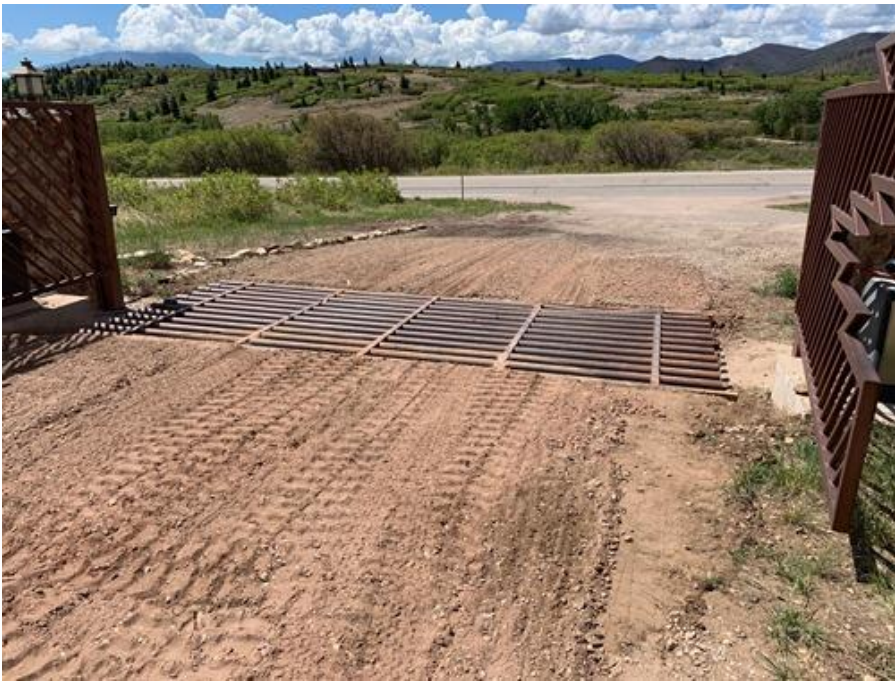
Cattle Guard after re-installation and regrading
